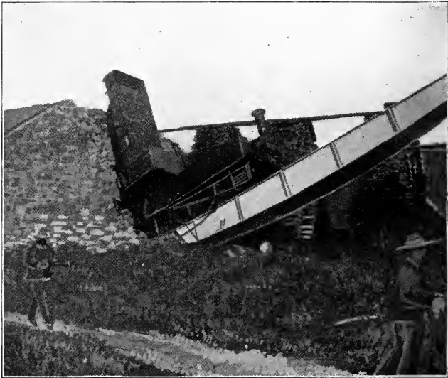
Side view of the Malelane Bridge, wrecked by British Scouts, sixty miles inside of the enemy's lines.
